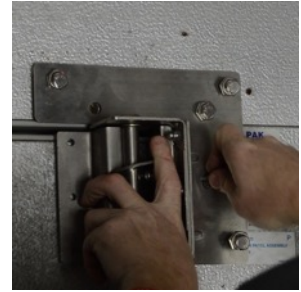
Figure 5: Tightening Expansion Bolts
