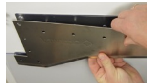
Figure 6: Attaching plates to PVC panels
