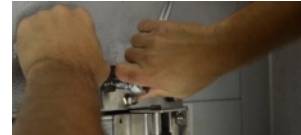
Figure 5: Tightening Expansion Bolts
